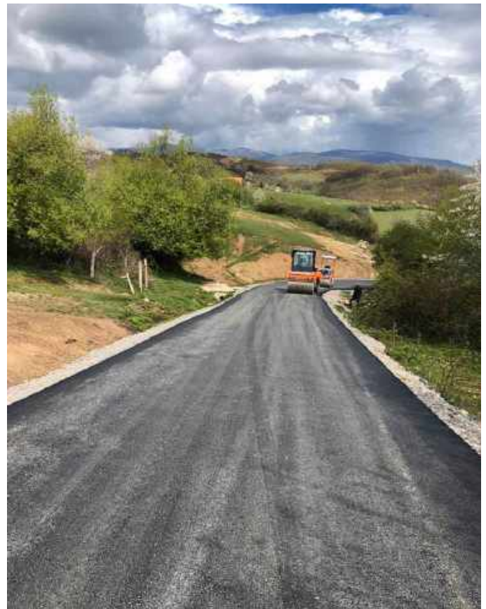
Figure 55. Improving road infrastructure Mitrovica South Municipality 2020
