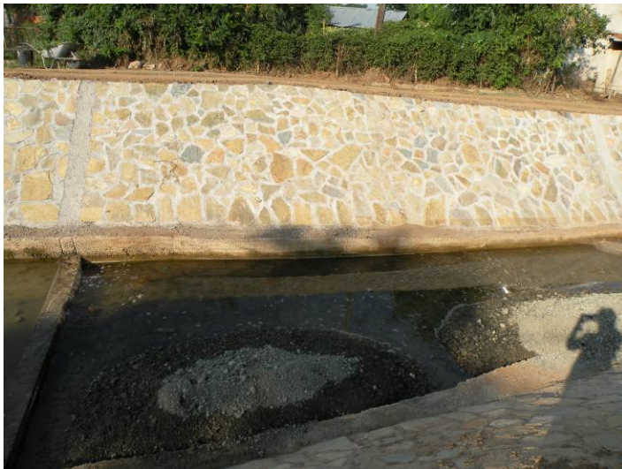
Photo No. 20: careless release of construction waste (gravel) into the newly regulated riverbed of the Gracanka River
