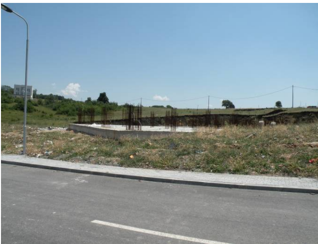
Photo No 7: The foundations of the new hospital near Susica
