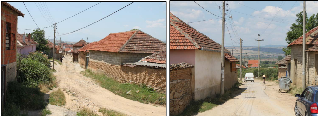
Figure 3.6.1 Poor road conditions are the main cause of dust in the dry season
