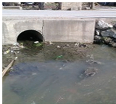
Photo 17. Running of wastewater into river
