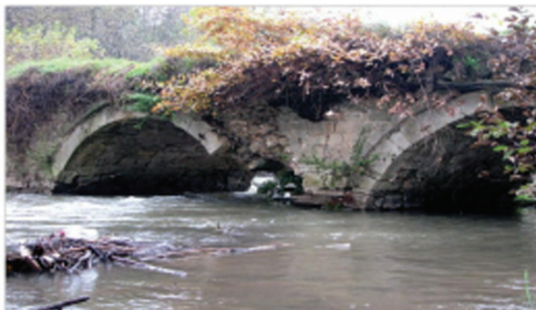
Picture 47. The Zallçi Bridge, before the restoration
