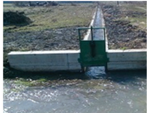
Picture 33. Water management (penstock)
