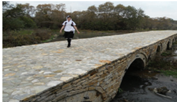
Picture 48 The Zallçi Bridge, after the restoration
