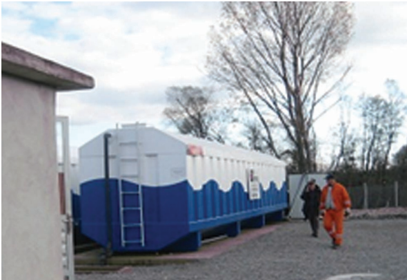
Picture 34. Waste waters treatment plant in Bajicë
