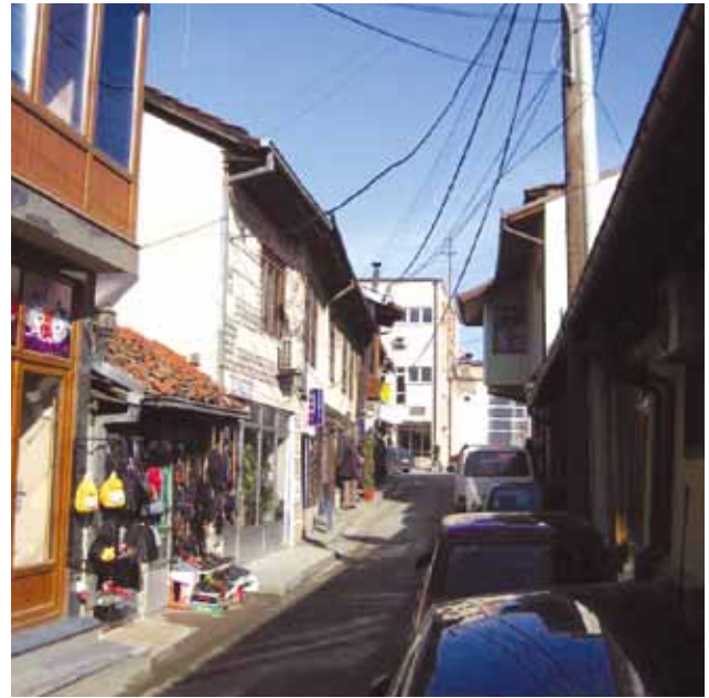
Project site 2: Before
