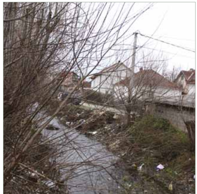
Project site 2: Before
