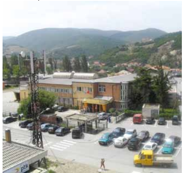
Project site 2: Before
