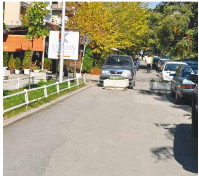
Project site 2: Before
