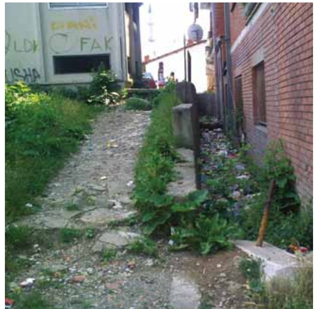
Project site 2: Before
